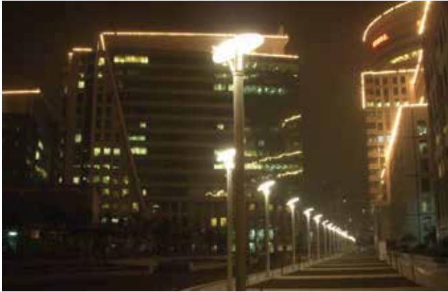
FYZT-8001 LIGHTING COLUMN at DLF Cyber City (Gurgaon)
