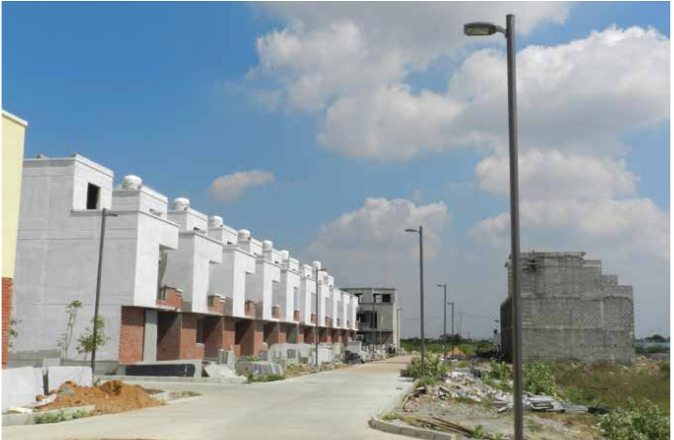
FYZD-797 Streetlight Lighting Column at DPS School (Chennai)
