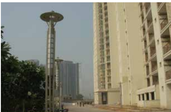
FLOATING Indirect Customise Lighting Column at DLF Summit (Gurgaon in 2008)
