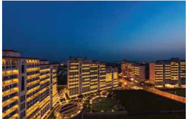
DURIN IP-65 Balcony Lights at DLF Skycourt
