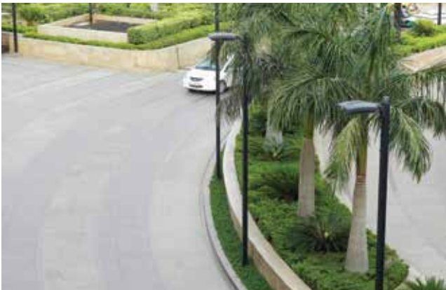
FYZD-797 STREETLIGHT at DLF Emporio Mall (Delhi)
