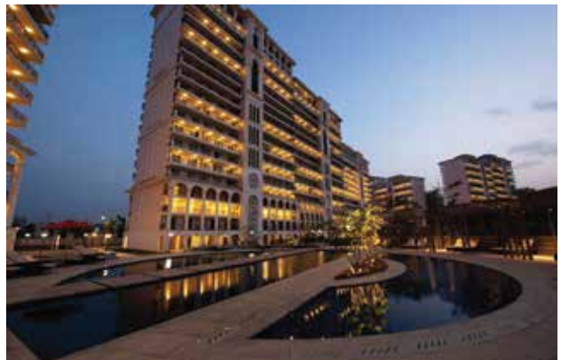
DURIN IP-65 Balcony Lights at DLF Skycourt
