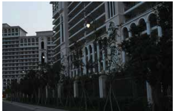
FYZT-501 at The DLF Skycourt, Sector-86 (Gurgaon)
