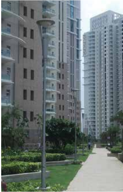
HOOD TL91-03 at DLF Park Place (Gurgaon)
