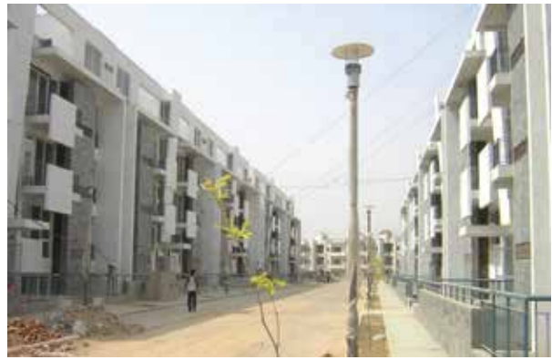
FYZT-8021 POST TOP at Vatika City, Sector-49 (Gurgaon in 2006)
