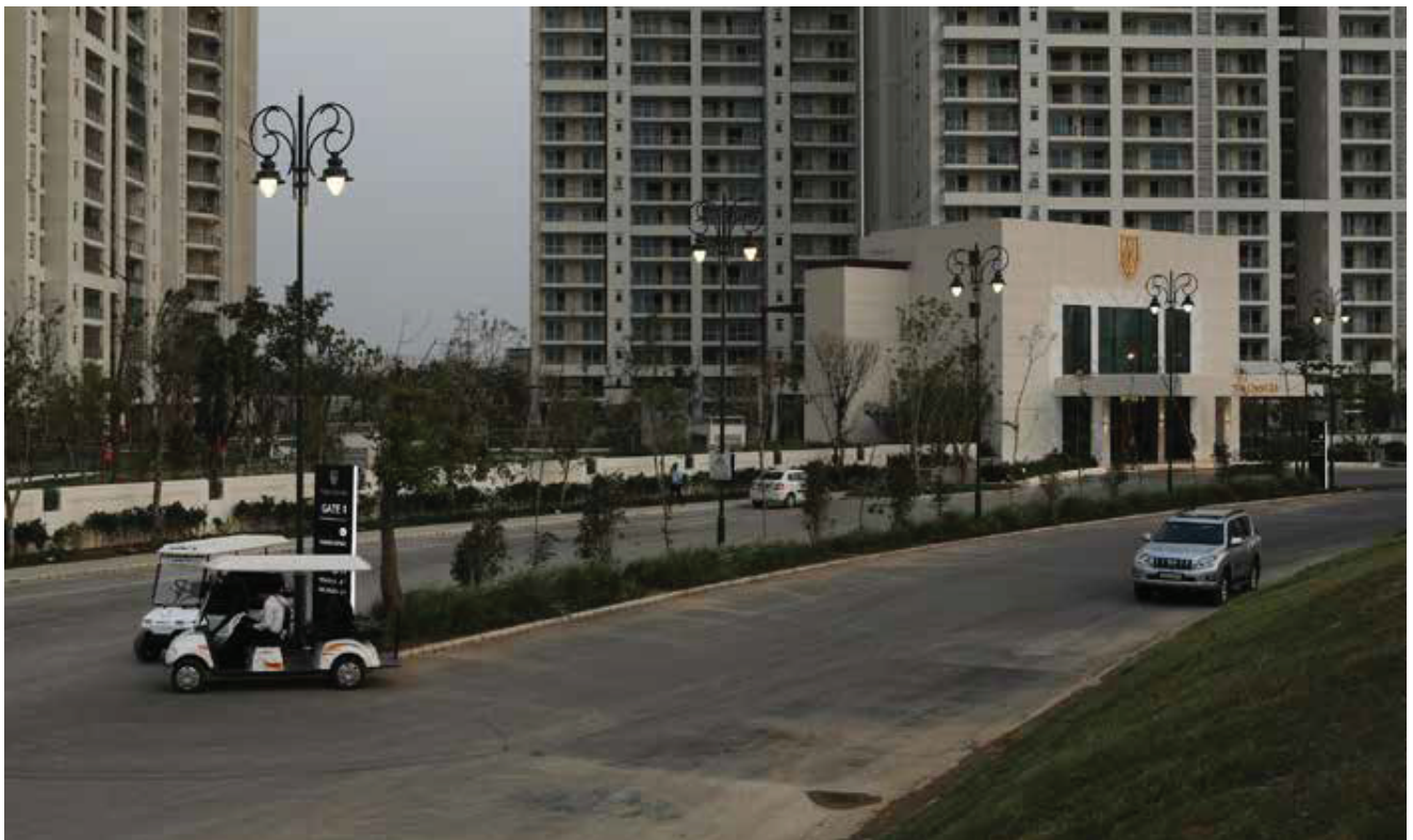
Dlf Crest, Gurgaon
