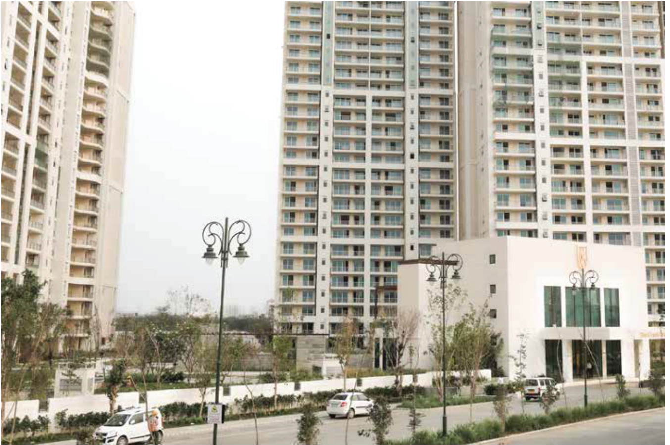
Dlf Crest, Gurgaon
